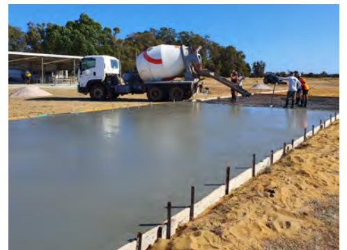
Second runway upgrade
