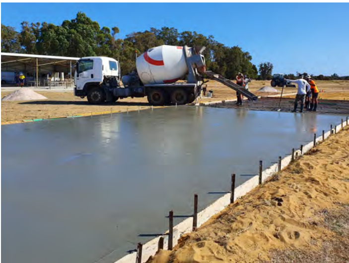
The completion of the second pour on the Northern end of the runway. Watered to slow the drying process.
