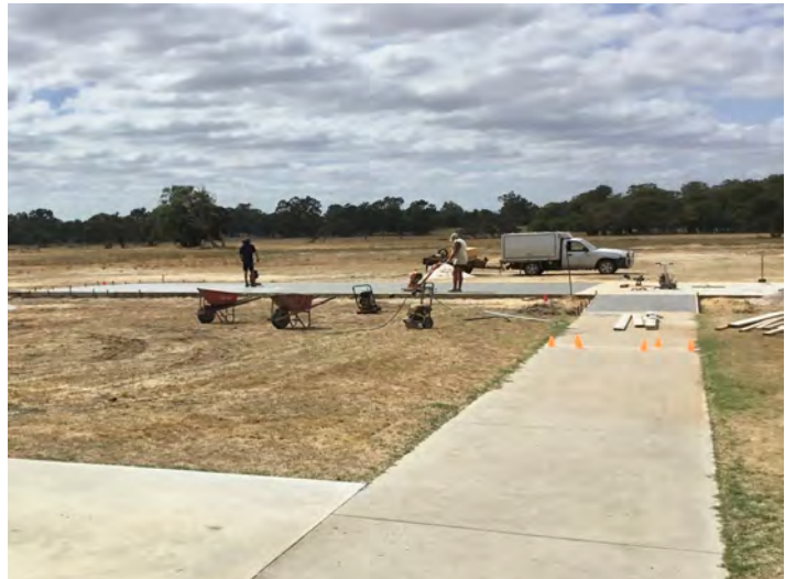
The Northern most end of the runway in final stages of completion the helicopter completing the surface finish. Project Completed just requiring back-fill now.
