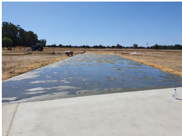
The completion of the second pour on the Northern end of the runway. Watered to slow the drying process.
