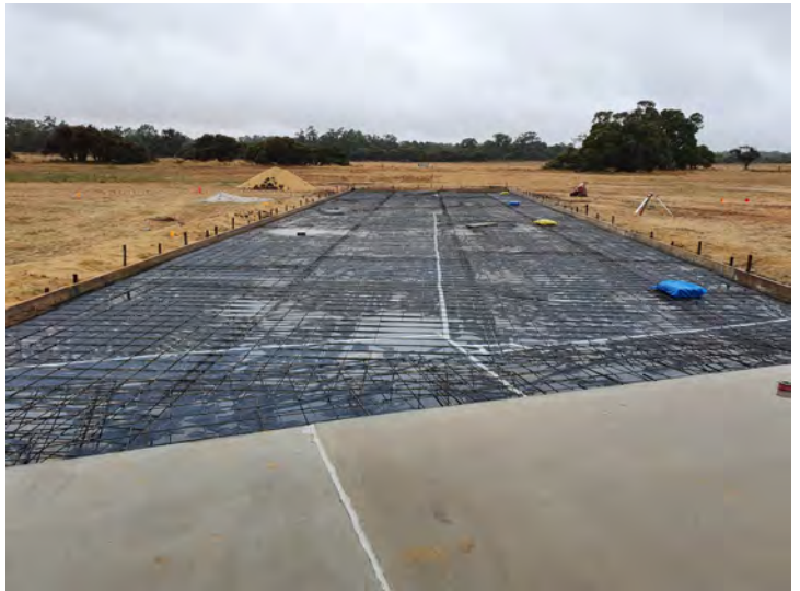
The expansion joints on the East/West runway were upgraded, the foam rubber was removed and new section inserted with Sikaflex.
